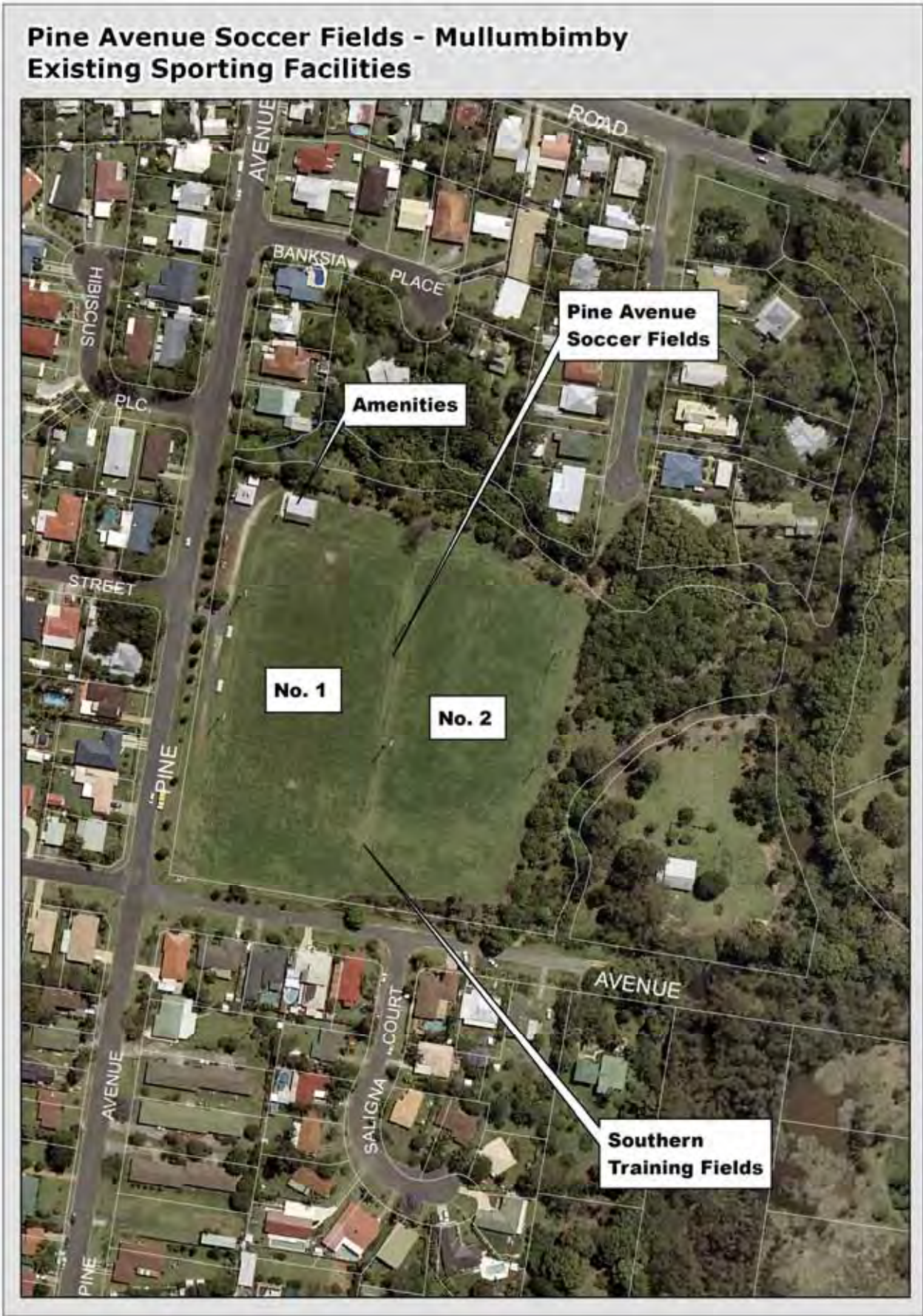
Figure 5 – Pine Avenue Soccer Fields - Mullumbimby
